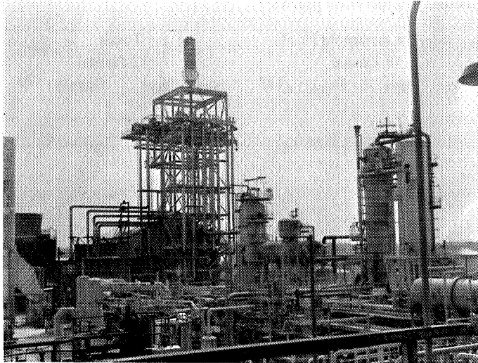
The M.W. Kellogg ammonia plant in Hopewell, Va.
